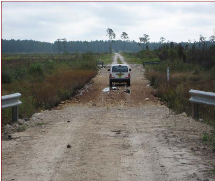
THSF Figure 2: A low-water hard-surface crossing installed on Deep Creek Road as part of the Doyle Creek Mitigation Project.
