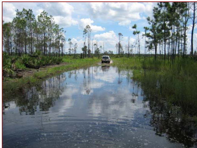
SSF Figure 3: Interrupted sheetflow on East Spur Road. Berm removal and installation of a hardened low-water crossing would enhance site hydrology and improve water quality.
