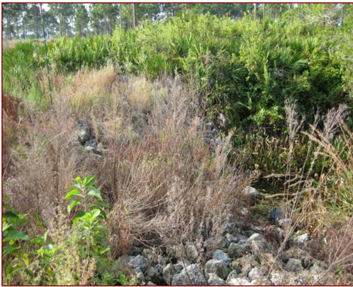
MSF Figure 1: Earthen/Rock ditch plug installed during the second phase of the Talon Bay Mitigation Project to restore hydrology to the forested wetlands.
