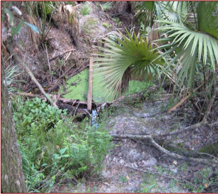
LBESF Figure 3: Spencer-Leeper ditch, which drains into the Econ River, shows signs of degradation and over-use from the bicycle and hiking trails on its berms. Erosion and sedimentation is impacting the flow in the ditch at places.
