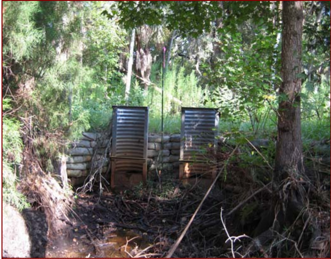
LBESF Figure 1: Flashboard risers installed as part of the SR 434 Mitigation Project on the Demetree Tract. At the time of the photograph conditions on the forest were very dry.
