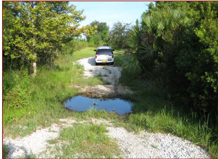
LBESF Figure 2: Low-water hard-surface crossing on the Demetree Tract. Surface flow through this crossing leads to the Econlockhatchee River.
