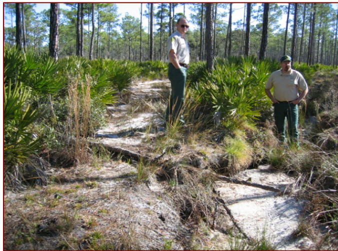
LWRSF Figure 3: Old forest roads and firelines on the Arbuckle Tract capture surface runoff and accelerate drainage which may alter wetland and unique plant communities on the forest.
