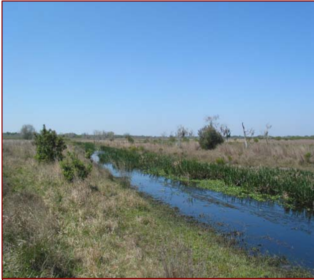
LWRSF Figure 2: Old ditch draining Otter Slough on the Prairie Tract. A fixed-elevation weir and elevated low-water crossings will restore the hydrology and hydroperiod of the site.
