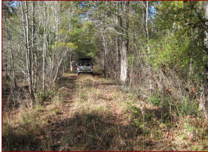
LTSF Figure 2: Above-grade woods road divides a natural drainage on the Searcy Tract. Installation of a culvert or low-water
