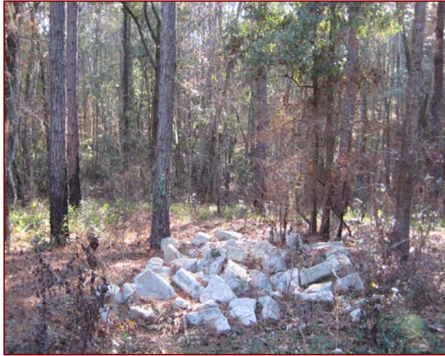
LTSF Figure 1: Rip-Rap “Apron” placed beside a dip in a service road at the top of a ravine on Rocky Comfort Tract. These structures are placed to protect against erosion and sedimentation into bottomland wetlands.
